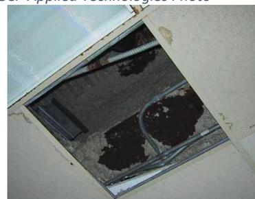
*SFRM or IFRM can be damaged when new services are added to existing buildings and need repair and documentation of the repair to comply. GCP Applied Technologies Photo*
