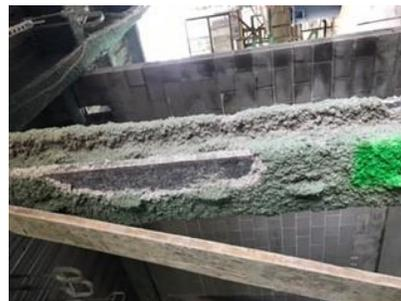
*SFRM or IFRM can be damaged during construction, then repairs are needed. GCP Applied Technologies Photo*
