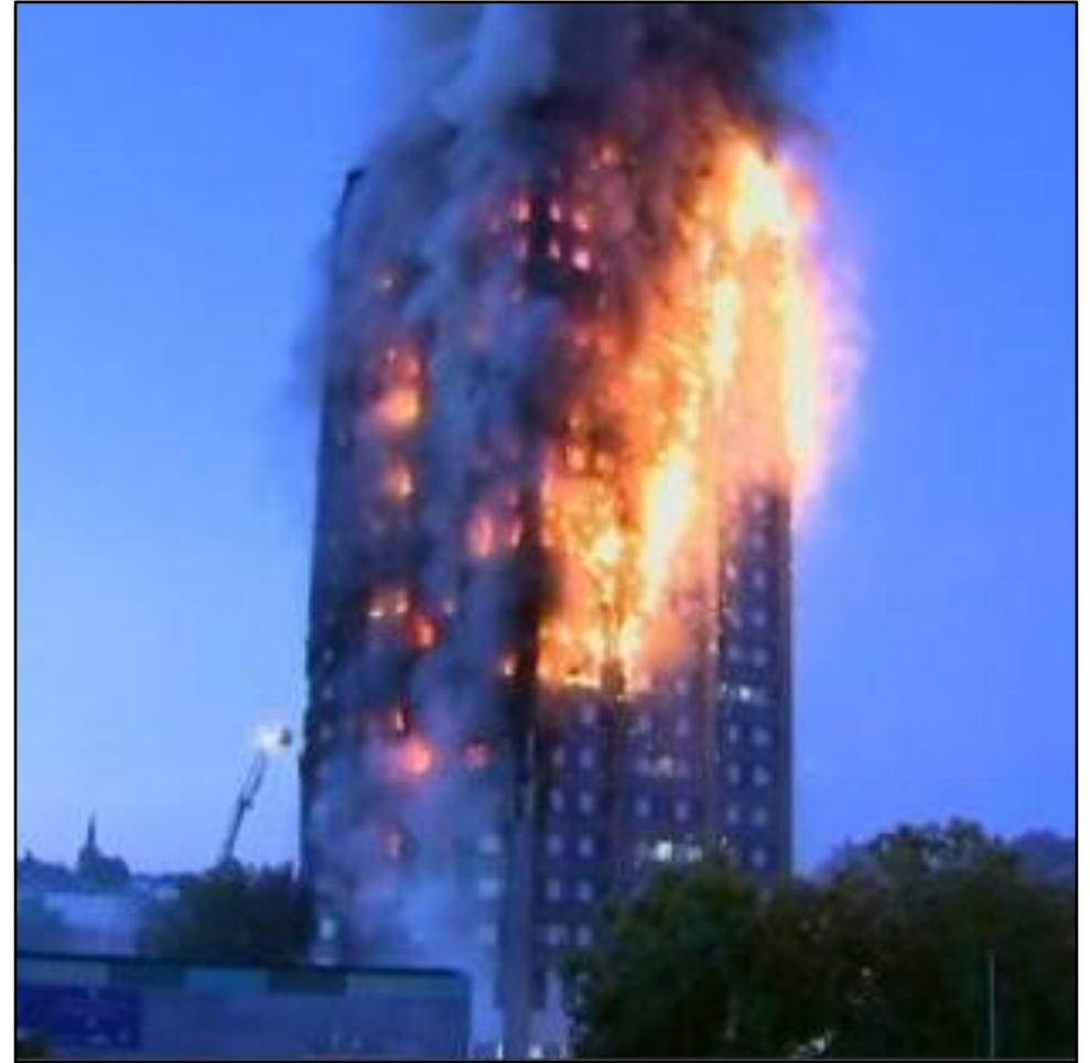
Grenfell Tower Fire – June 14, 2017
