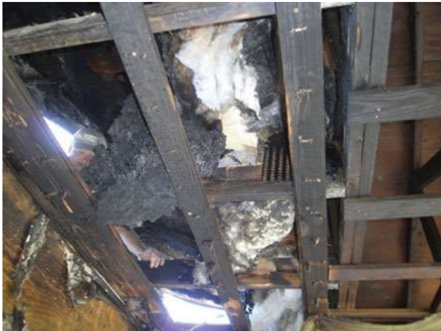
Four examples of fire damage from exothermic ignition from an excessive amount of foam applied in a single pass to fill and seal the soffit area. PHOTOS PROVIDED BY MASON KNOWLES
