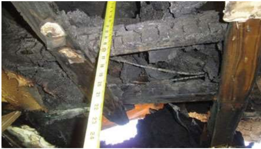
Four examples of fire damage from exothermic ignition from an excessive amount of foam applied in a single pass to fill and seal the soffit area. PHOTOS PROVIDED BY MASON KNOWLES
