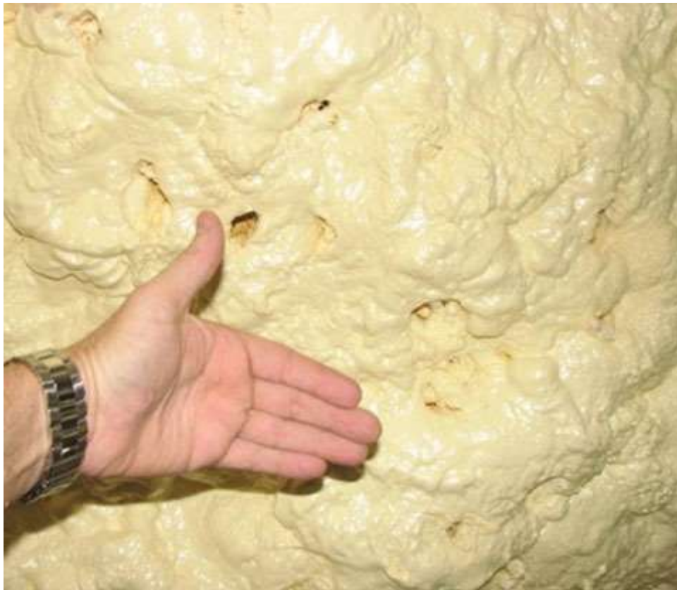
Voids caused by exceeding the recommended lift thickness. PHOTOS PROVIDED BY MASON KNOWLES
