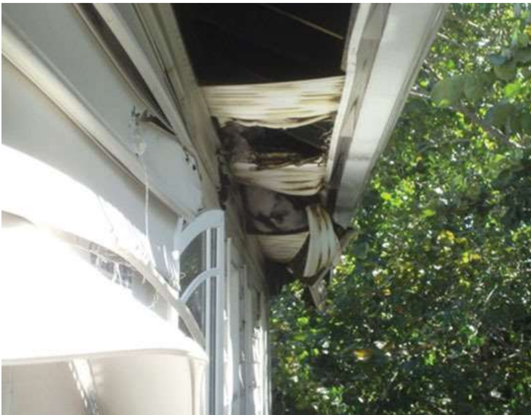
Four examples of fire damage from exothermic ignition from an excessive amount of foam applied in a single pass to fill and seal the soffit area. PHOTOS PROVIDED BY MASON KNOWLES
