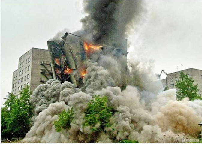
An apartment block in St Petersburg, Russia (2002) Reinforced concrete: FULL COLLAPSE
