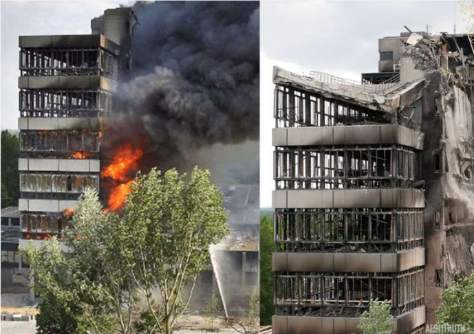
Delft University, Netherlands (2008): Steel concrete hybrid: PARTIAL COLLAPSE
