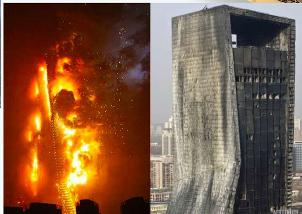
Mandarin Oriental Hotel/Beijing Television Cultural Centre in Beijing, China (2009): NO STRUCTURAL DAMAGE OR COLAPSE
