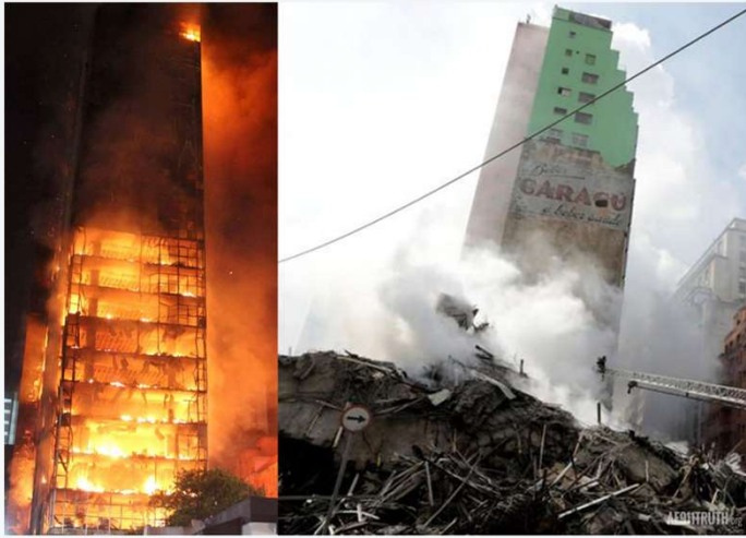
Wilton Paes Almeida Building in São Paulo, Brazil (2018): Concrete & steel building: COLLAPSE
