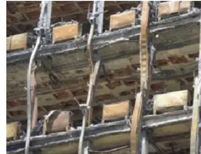
Buckling at floor 9
